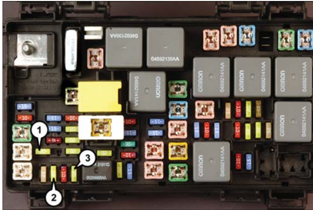
Power Outlet Fuses
